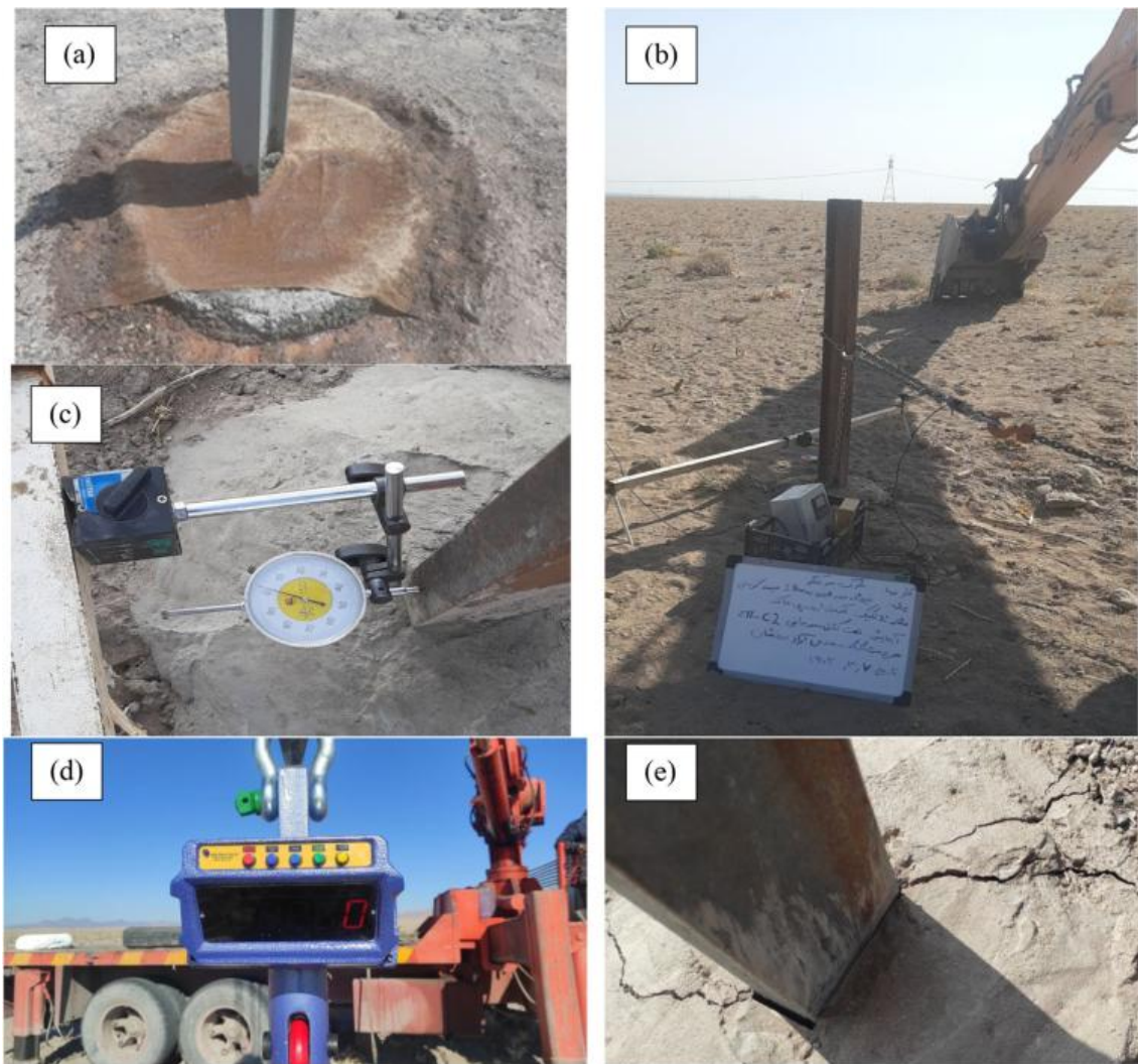
Fig.3 (a) Preparation of concrete pile (b) Lateral loading (c) LVDT (d) Loading system (e) Failure moment of piles
